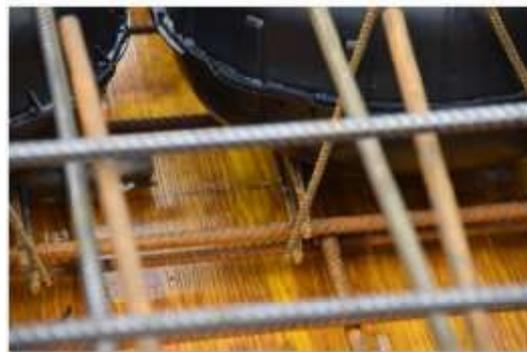
For the **“Alte Holstenstraße 59” project**, Heinze Cobias Deutschland GmbH delivered fixing elements which have been increased in height by 2.0 cm, so that the prefabricated void former modules were adapted to the specified slab depth.
