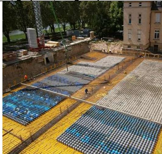
Cobiax void former modules installed prior to the concreting of the roof slab during construction of the underground garage for the Mannheimer Klinikum, which was subsequently turned into a green roof
