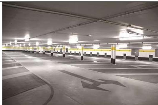
Interior view of one of the two parking levels in the underground garage at the Mannheimer Klinikum. This photo clearly shows that the individual parking spaces are free of columns, and that the underside of the slabs form a continuous level which is extremely installation-friendly for all building technology systems.
